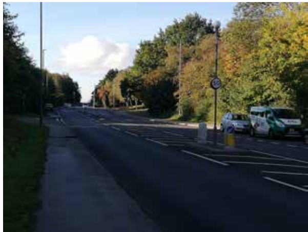
Facing south west along Coventry Lane
